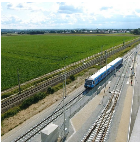
Wallersdorf – Rail siding
